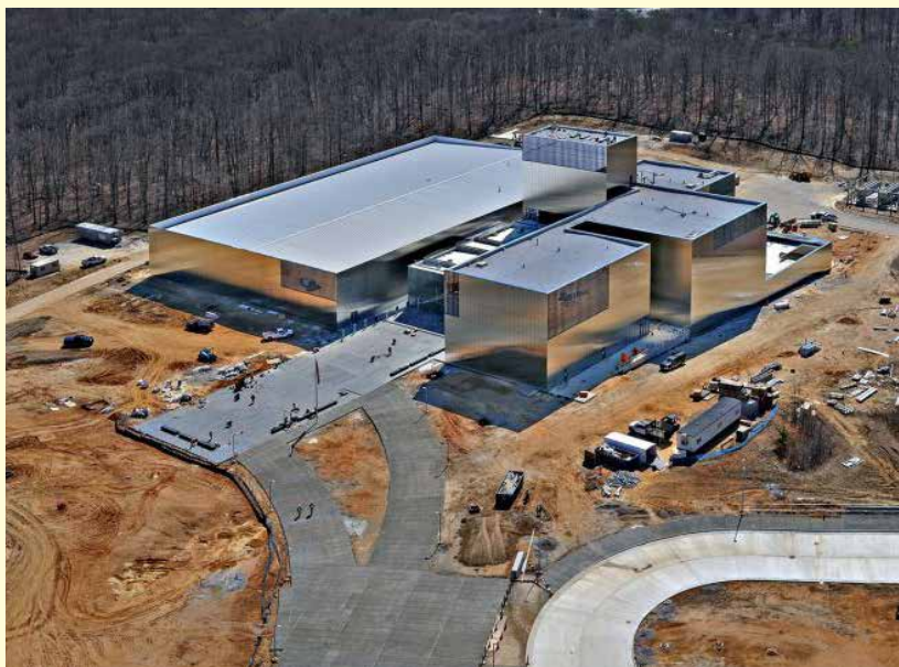
Museum under construction, as of March 2019
