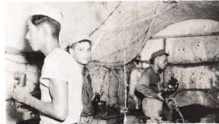
Okinawa Invasion—Underground Clean-up
